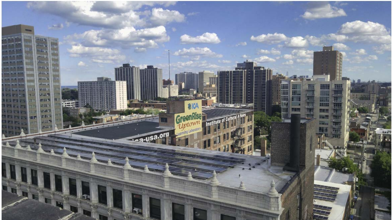
ROOFTOP SOLAR ARRAY
